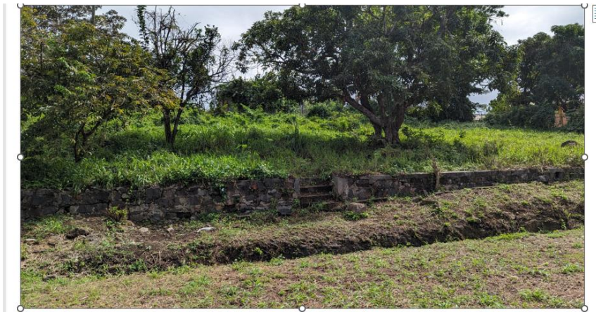
Image 2: Eastern boundary of the site along the masonry wall (Eastern end)
