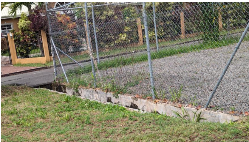
Image 3: Concrete Box drain along NADMA Premises (Northern end)
